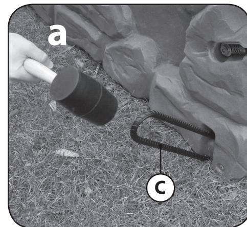
**Hammer the Anchor (C) in at a 45 degree angle on opposite corners.**
